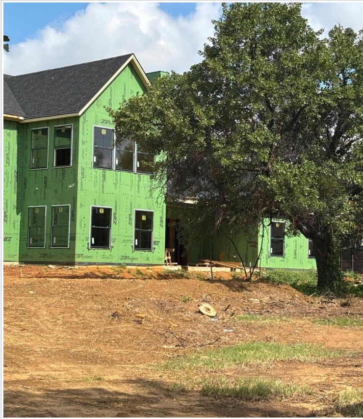
Grade change 1 — raised building pad and exposed slope near the house.
