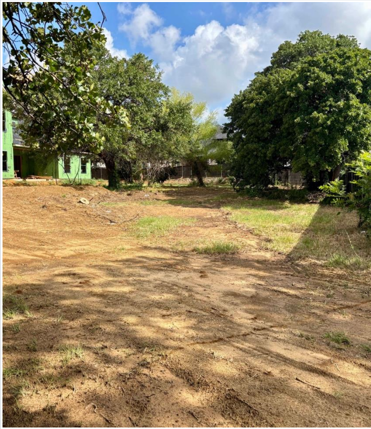
Runoff 1 — broad disturbed surface and apparent channel through the yard.
