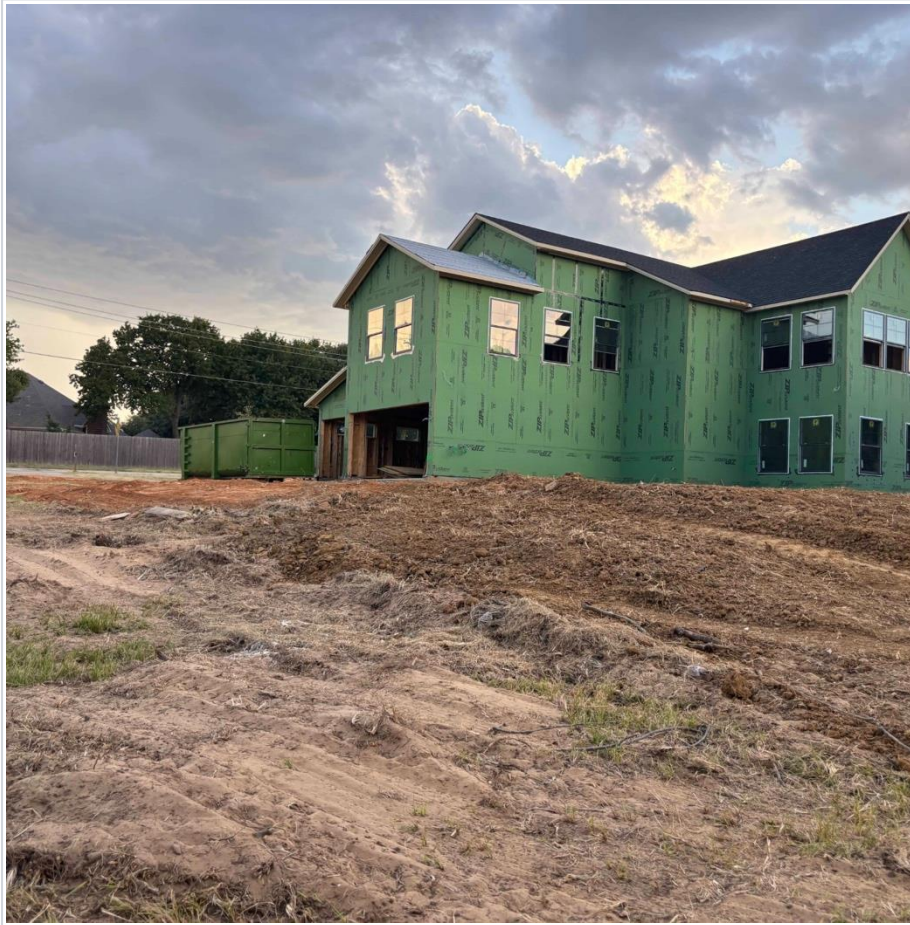
Grade change 4 — raised pad and fill adjacent to the new structure.
