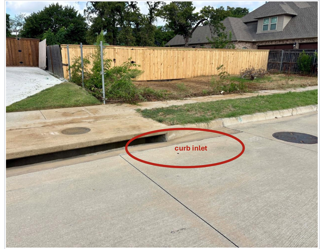
Runoff 6 — nearby curb inlet / municipal storm-drain entry.
