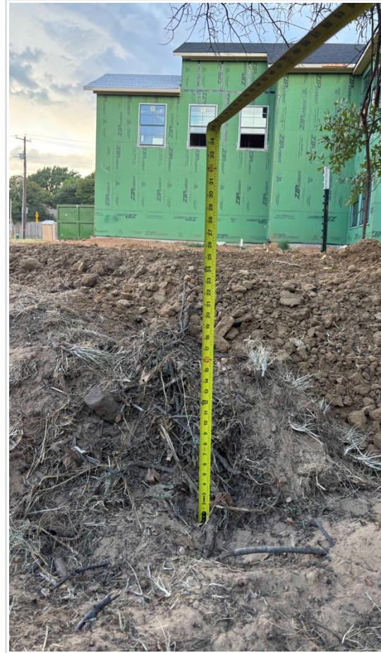
Grade change 5 — 26" of dirt added.
