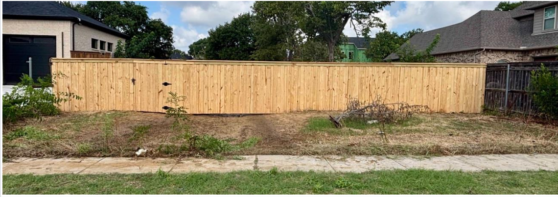
Runoff 4 — street-side fence and disturbed soil behind it.
