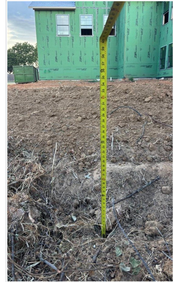
Grade change 6 — 34" of dirt added
