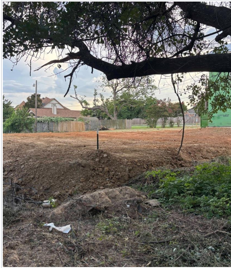
Grade change 2 — broad disturbed area with fill and altered surface contours.
