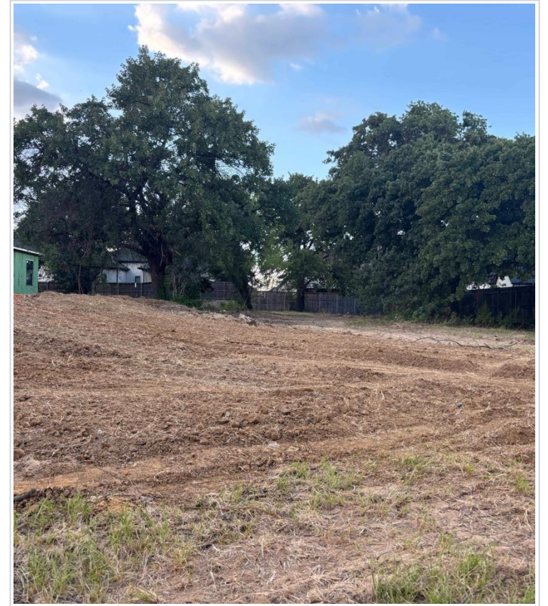
Grade change 3 — visible fall from the building pad toward the side/rear yard.
